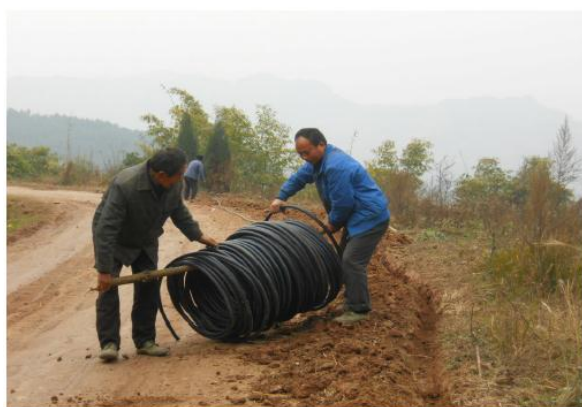
Qinggangping villagers setting up water pipe
