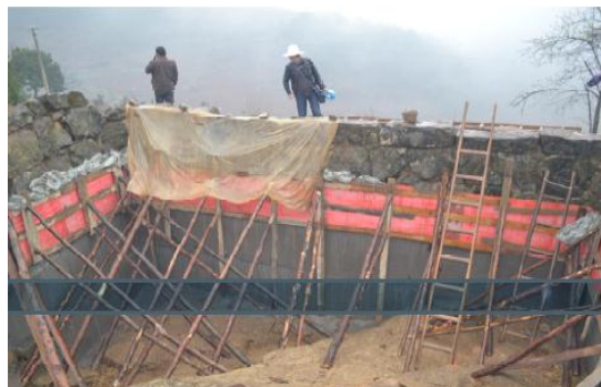
Drinking water tank construction
